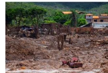
Brumandinho dam collapse (Brazil, 2019)
